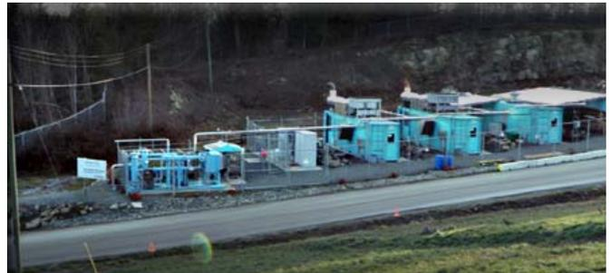
The 1.3MW facility became operational in March 2009 and is currently operating at half capacity due to a constricted supply of landfill gas. As part of a larger improvement to the landfill completed in June 2010, the RDN has extended the landfill gas collection field. The upgrade will increase the capture of landfill gas allowing Cedar Road LFG Inc. to increase the supply of electricity it sells to BC Hydro and further reduce emissions.
